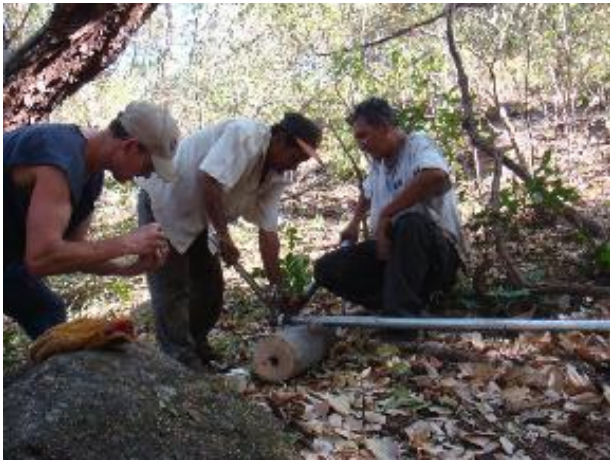
Above: Pedro and Pedro (two guys in white) from JHC working on tightening a coupling while Bucknell professor Mike Toole (in blue at left) cleans the next elbow for installation.
