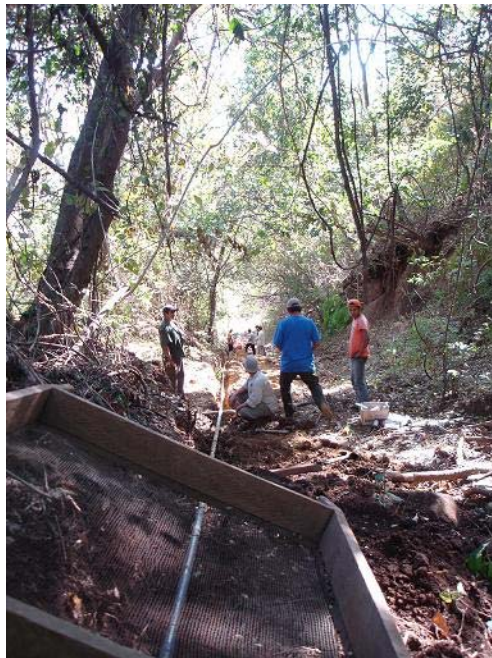
Above: Pedro and Pedro (two guys in white) from JHC working on tightening a coupling while Bucknell professor Mike Toole (in blue at left) cleans the next elbow for installation.
