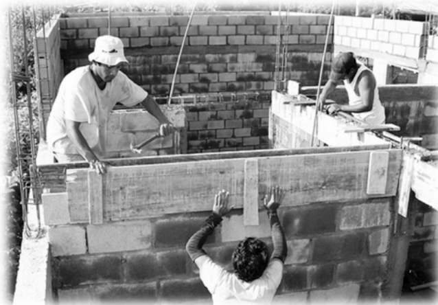
Community members build the Monte Horet Pre-School, funded by PGL
